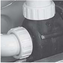
Vent air by slightly opening pump unions.
